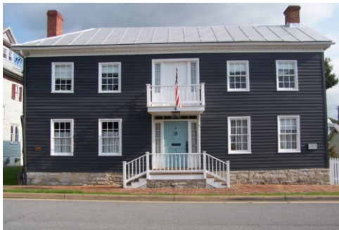
Blazer Huber House - 148 West King St.
