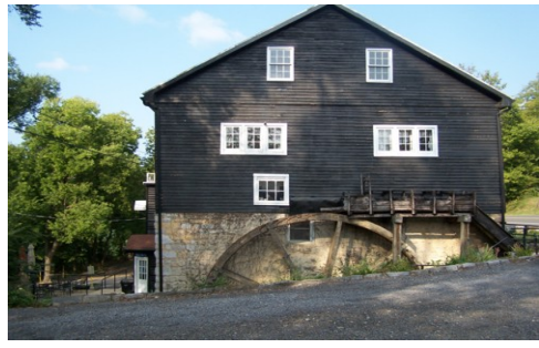
The Old Mill - 499 Stover Avenue
